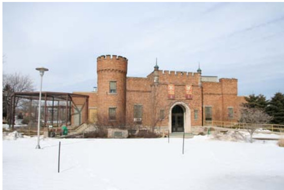
Racine Zoological Gardens Administration Building, 2129 North Main Street
